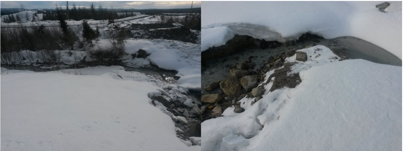
Figure 8. Dam overflow. Contact immediately Yara's specialists depending on the size of the flow or follow the emergency instructions.
