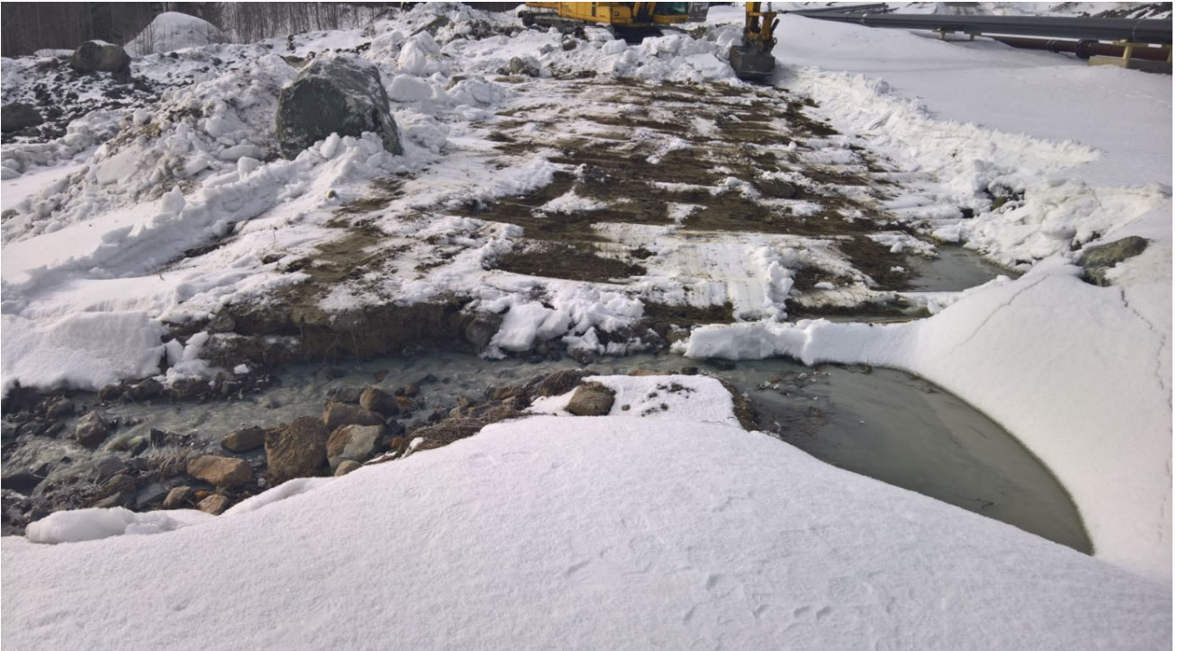
Figure 7. Dam overflow. Contact immediately Yara's specialists depending on the size of the flow or follow the emergency instructions.
